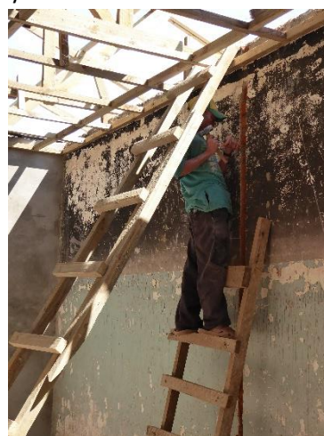
Refurbishing the dormitories at Idodi
